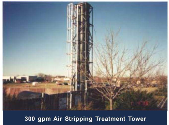
Tower Modification and Reconstruction
